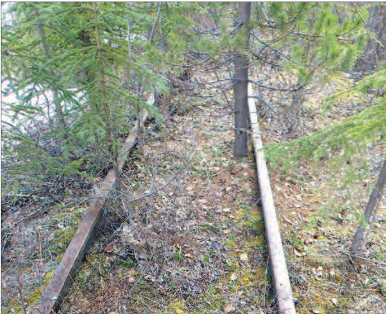
A SERIOUS OBSTACLE – A significant tree is growing up between the rails near Mary Lake.
